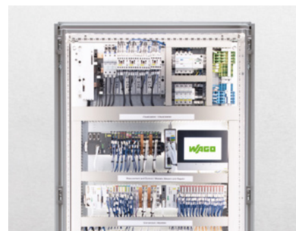
Classic: Installation of automation components in the control cabinet
