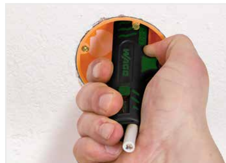
Stripping a cable sheath.
