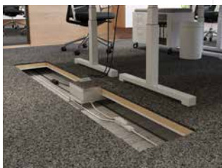
Installation of Underfloor Systems
